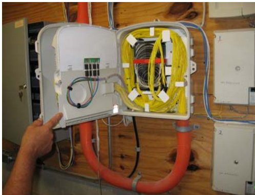
FIOS fiber optic cable installation
