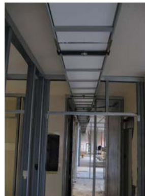
Open ceiling office tray
