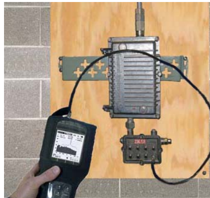
Field testing of signal levels using a meter
