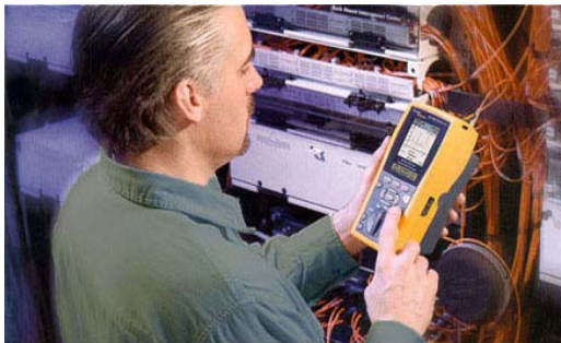
Fiber optic cable certification
